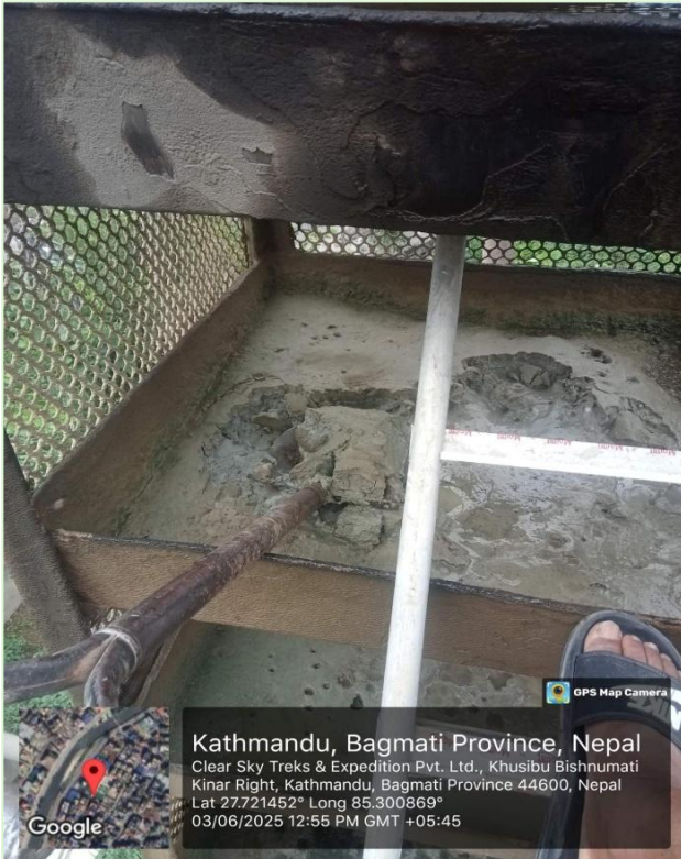
Fig: Filter Media wash at Khusibu Water Treatment Plant.
