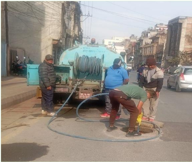
Fig: Sewer cleaning work at Kuleshwor and Jawalakhel
