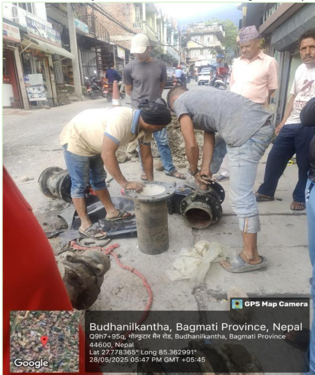
Fig: Leakage repair works were carried out near Budhanilkantha Mandir. The area had been experiencing frequent leakages, and the completion of this work has reduced inconveniences for local residents while also minimizing the risk of accidents
