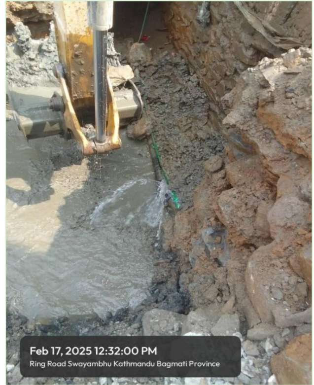
4" Dia. Pipeline Maintenance work at Thulovarang.
