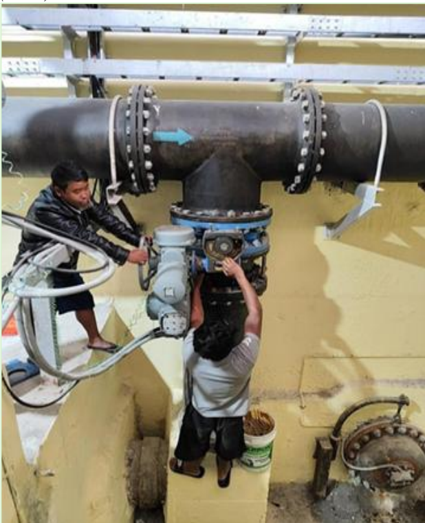
Fig: Servicing & Greasing of Valves
