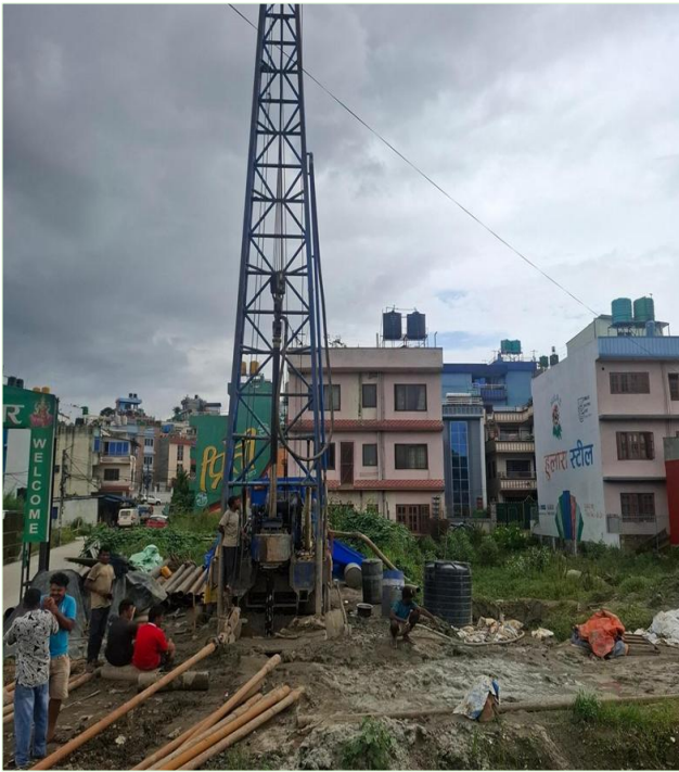
Fig: Drilling of new well at Gothataar
