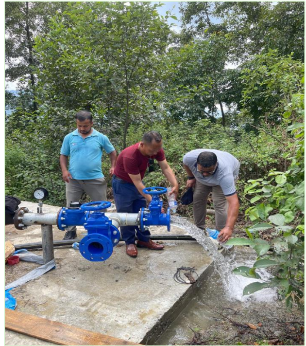
Fig: Operating new well at Changunarayan
