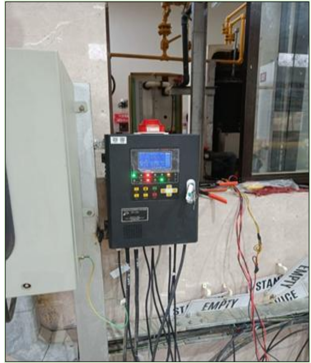
Fig: Installation of Chlorine leak detector (CLD)
