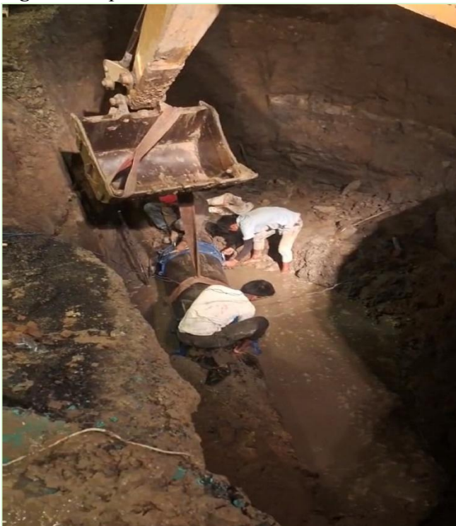
Fig: Joining of pipe and Mechanical Coupling at Pulchowk
