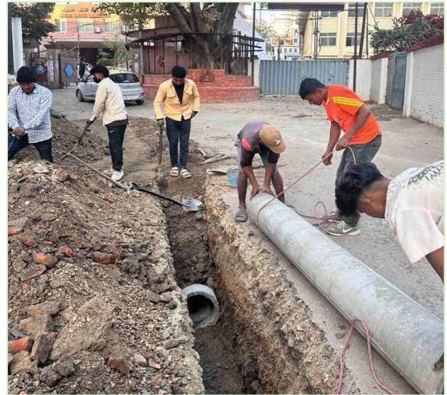
Fig: New sewer construction work at Kupondole (Rio Marga) & Anamnagar
