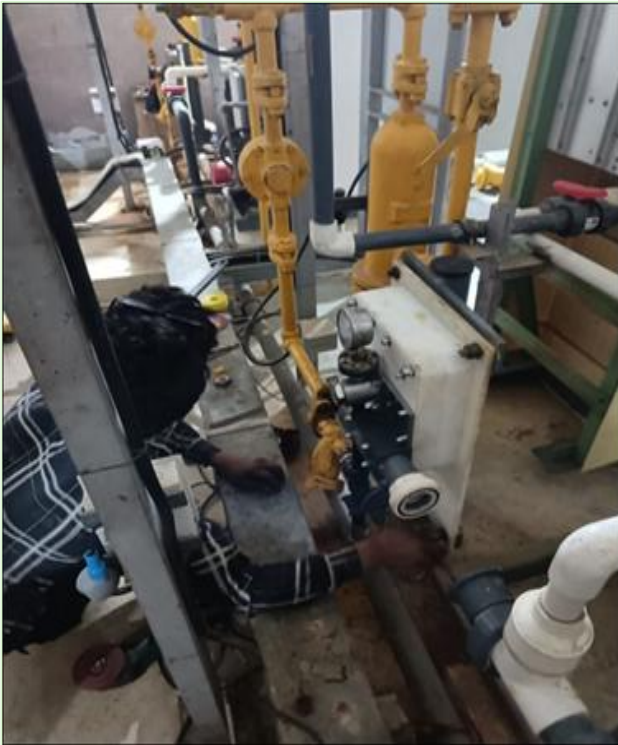
Fig: Installation of Remote vacuum regulator (RVR)
