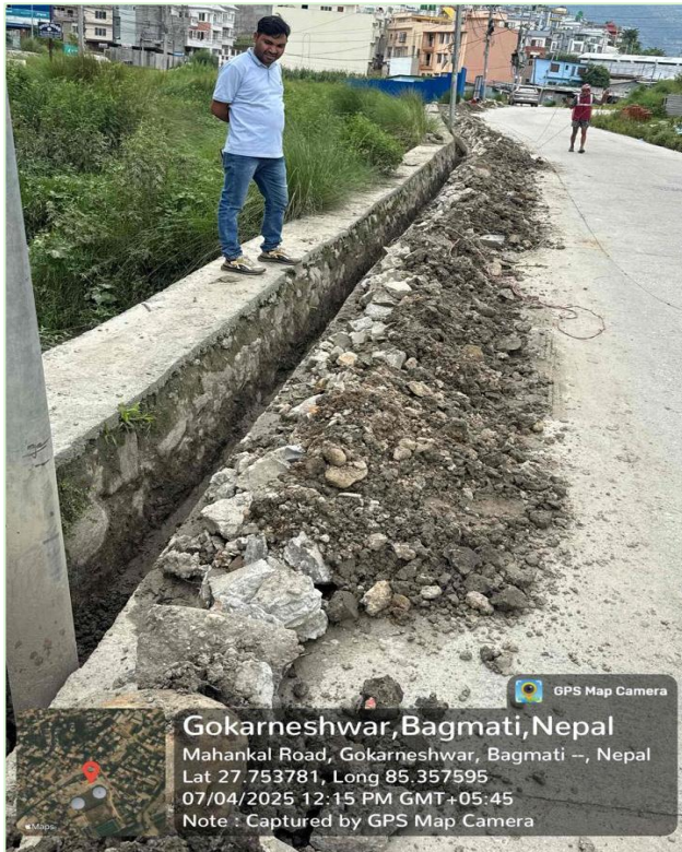
Fig: For increasing service area, 4" HDPE pipeline was extended in the Bhangal area. This pipeline has enabled the connection of 200 households that were previously not integrated into the water supply network.
