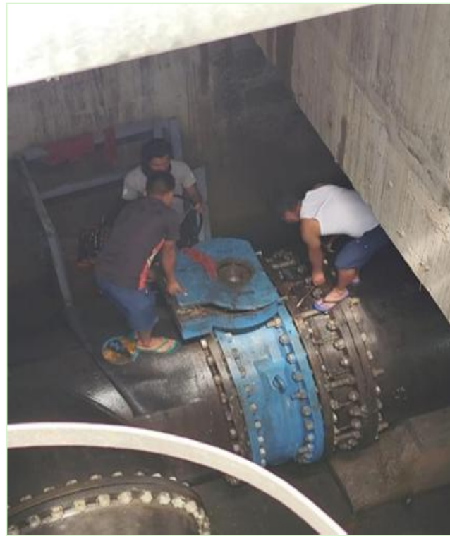
Fig: Servicing & Greasing of Valves
