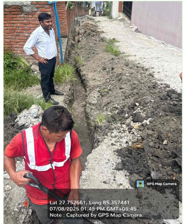
Fig: For increasing service area, 4" HDPE pipeline was extended in the Bhangal area. This pipeline has enabled the connection of 200 households that were previously not integrated into the water supply network.
