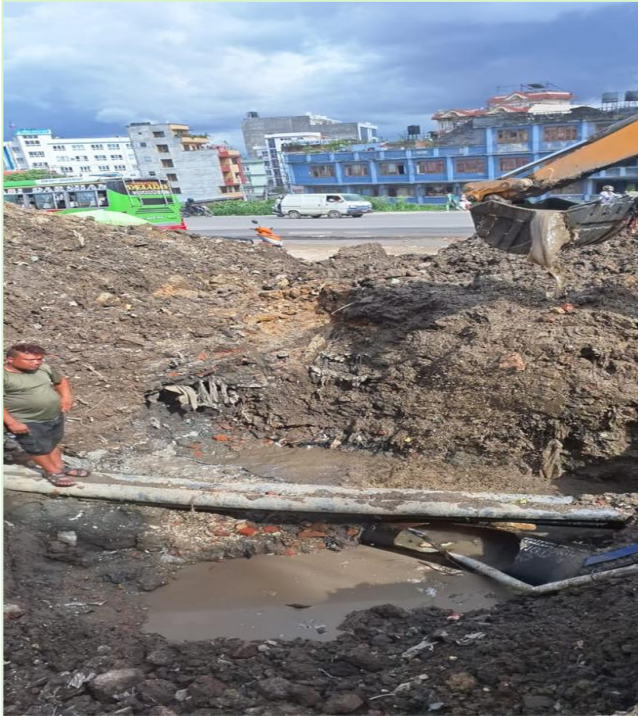
Fig: BDS repair at Banasthali
