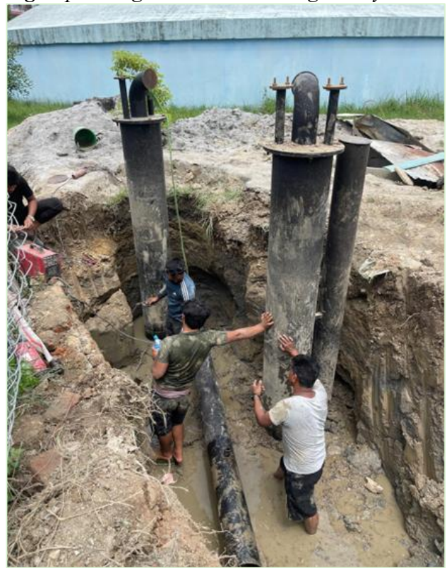
Fig: Construction of new sumpwell for Kapan Supply
